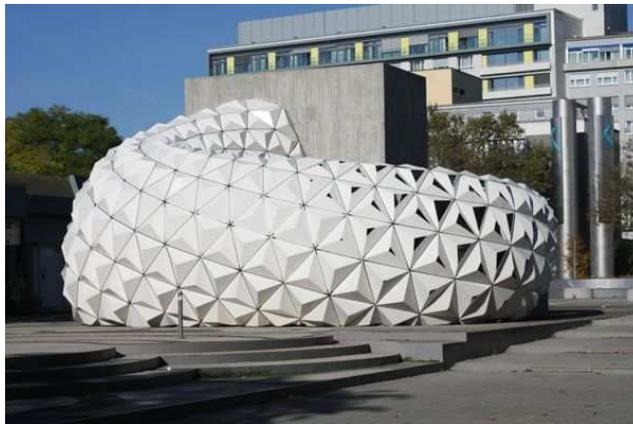
Figure 3: Bioplastic facade mock-up
